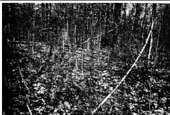
Figure 8-6 Collapsed Pipe Tower at Peavine Mountain
