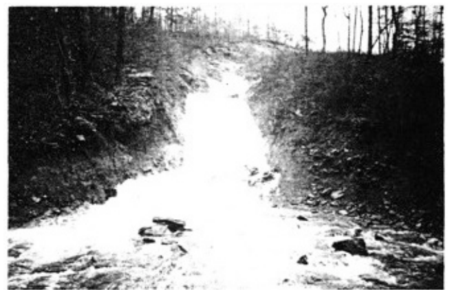
Figure 3-8 Glostowbury Spillway from the Bottom
